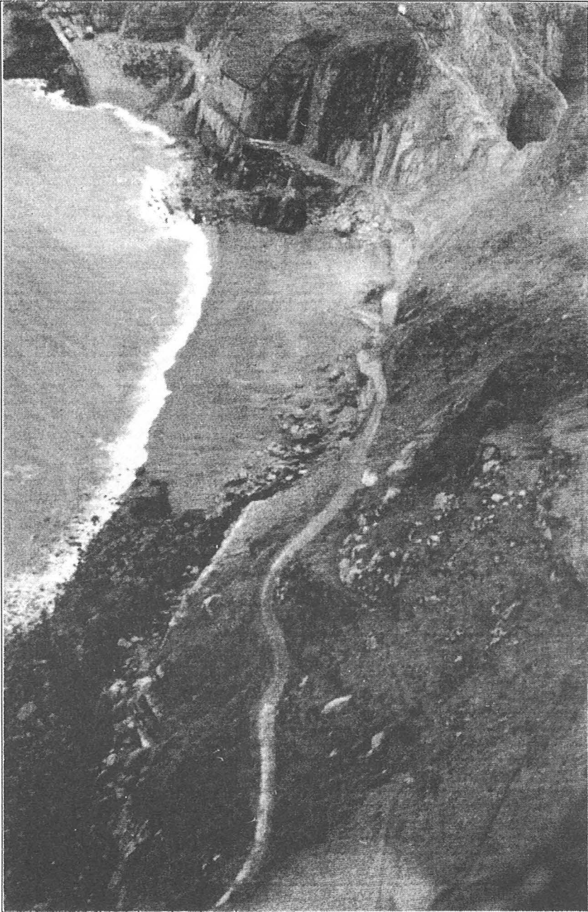
Plate 2: Divers Beach and Landing Beach 1998 prior to the start of the works.
