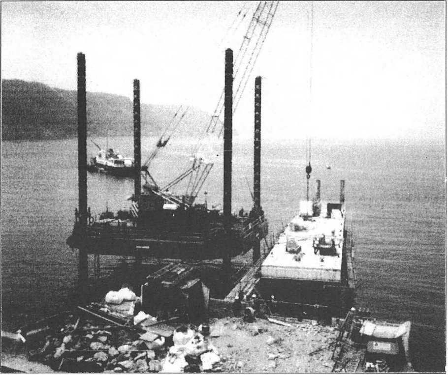
Plate 3: The jetty under construction July 1999.
