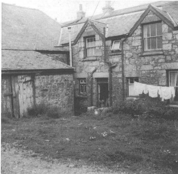
Figure 12. The backyard (north) of the Hotel in 1960. The door to the boiler room is open. (photo: M. Ternstrom)
