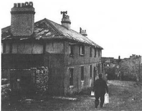
*Many of the houses on Lundy are badly dilapidated as the result of furious gales from which the island is unprotected. Slates are frequently torn from the roofs.*
